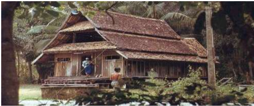
Figure 8. An example of creating a house in Southern of Thailand to live with comfortably under Thai wisdoms and setting the direction for the building in accordance with the sun and wind direction. (Search on; http://www.baanjomyut.com/library/thaihouse/ , February, 17, 2015)
