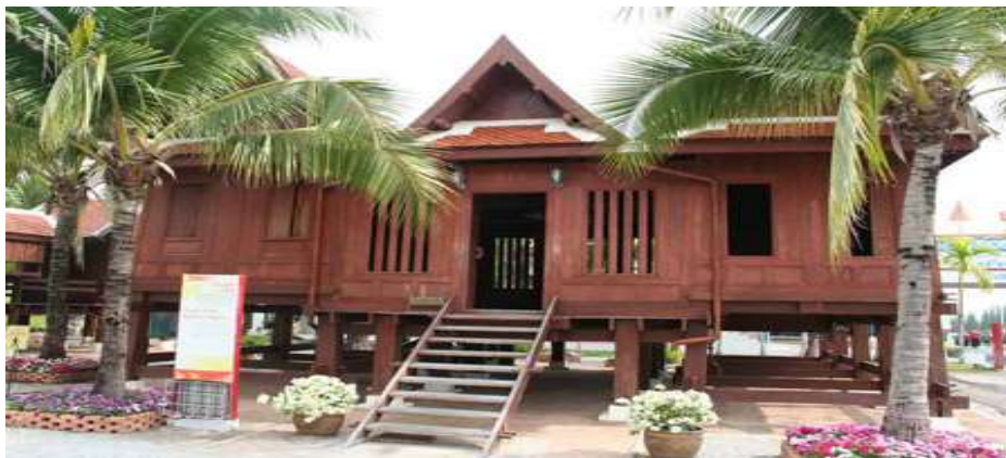
Figure 9. An example of creating a house in Southern of Thailand to live with comfortably under Thai wisdoms and setting the direction for the building in accordance with the sun and wind direction. (Search on; http://www.baanjomyut.com/library/thaihouse/ , February, 17, 2015)
