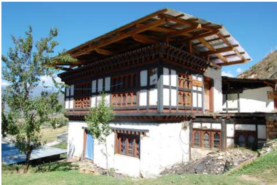
Figure. 3. The traditional architecture of housing in Bhutan is a 2 storey house, on an attic floor for stored agricultural crops, residential area use on the second floor, and the ground floor for horse, cattle or sheep stables, and farming tool. (Photo; Kitipong Tepjitara, Paro city, October, 12, 2013 )
